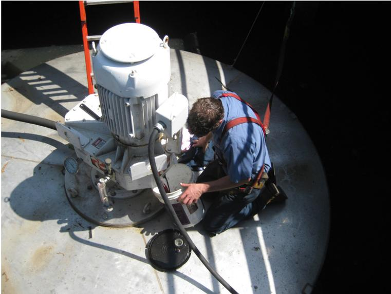
Jamie Piangerelli is seen here draining out the LE gear lubricant that the units were initially filled with.
