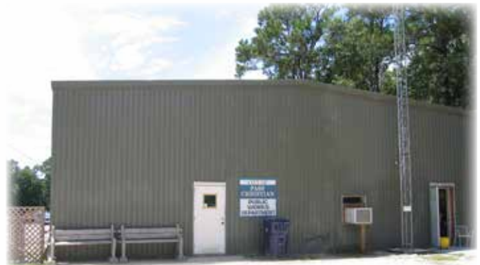
Pass Christian office and shop
